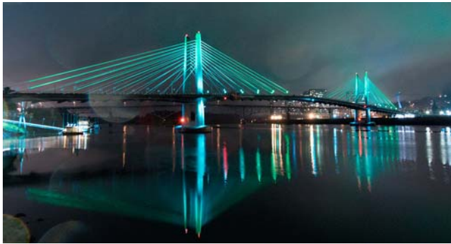
Tilikum Bridge, started by the Caruthers Crossing Rail Study, 1997.
