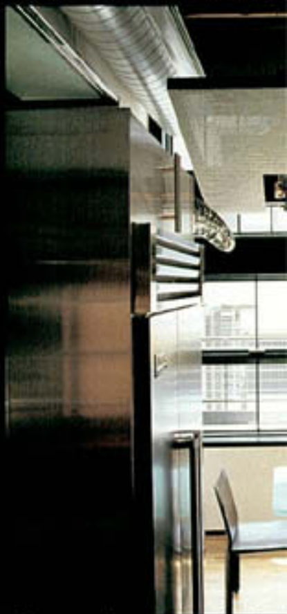
A hip-cut stainless steel mesh canopy hangs customized for the Del Castelllos' center isle
