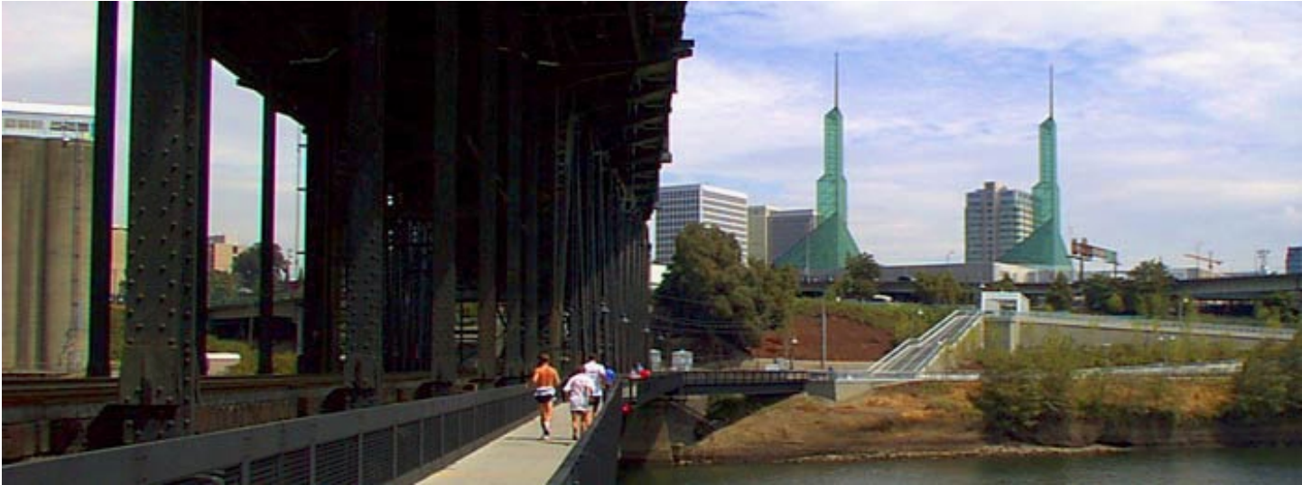
Pedestrian Walk at Steel Bridge with the Convention Center in the Background
