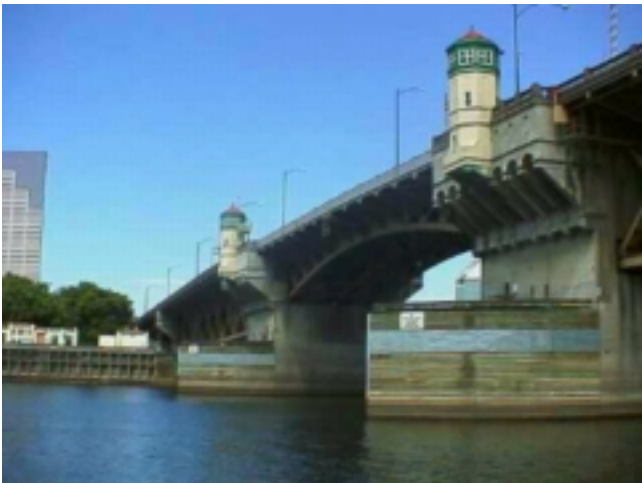
View of Burnside Bridge from Walkway
