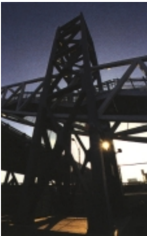
Access Tower to Burnside
