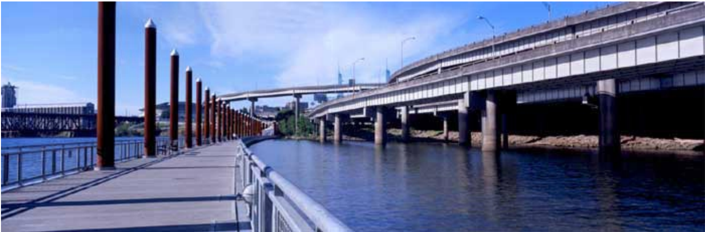
Floating Walkway along Interstate-5
