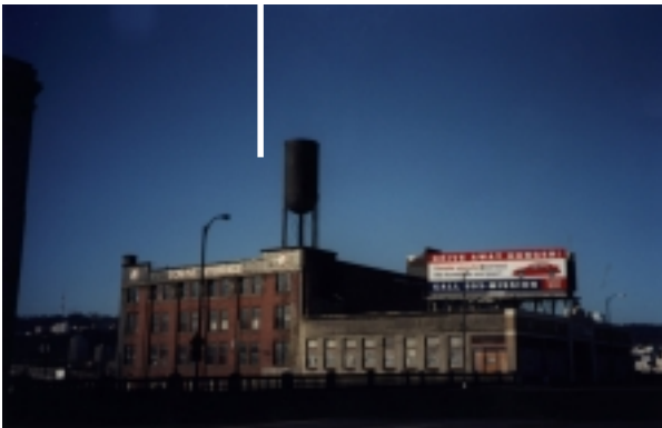
Towne Storage Building
